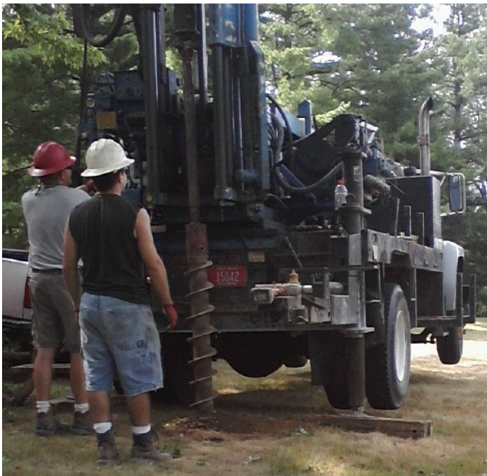
Figure 1. Well MW2B being drilled north of Clear Lake with the Wisconsin Geological & Natural History Survey drill rig.
