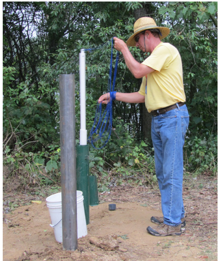
Figure 2. Development of well MW1B using a bailer.
